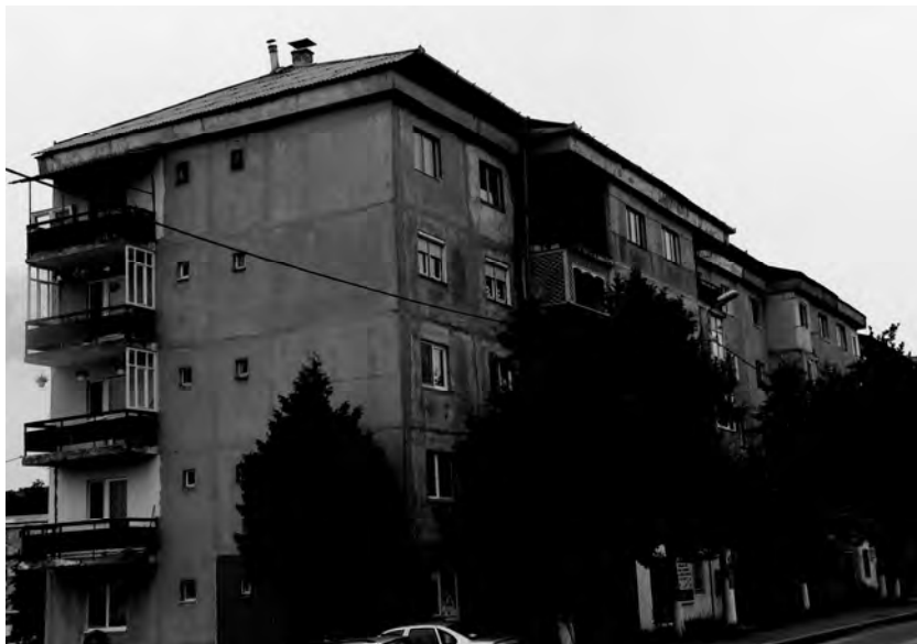
Figure 5. The apartments to be rehabilitated
