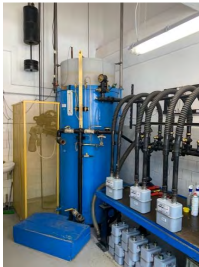
Figure 3. Installation of checking gas meters with bell
